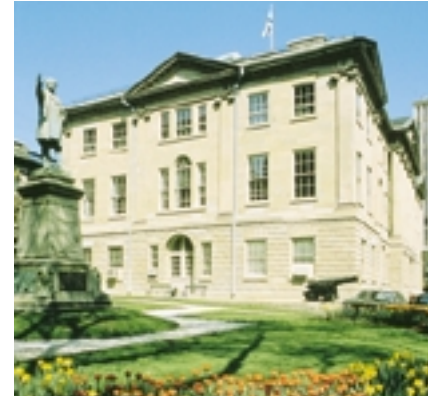
Figure 4.40B After sandblasting
